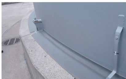
Tank bottom seal
