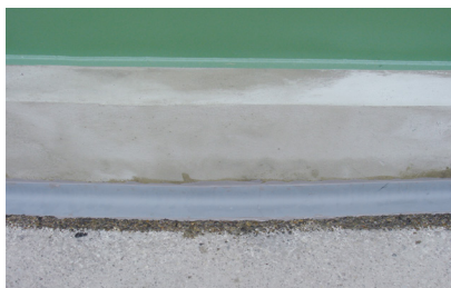
Tank foundation seal
