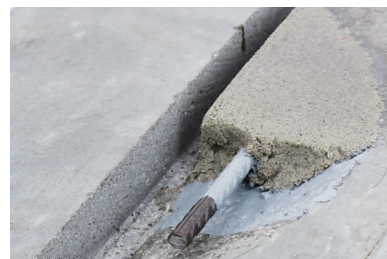
Manhole pit rim repair
